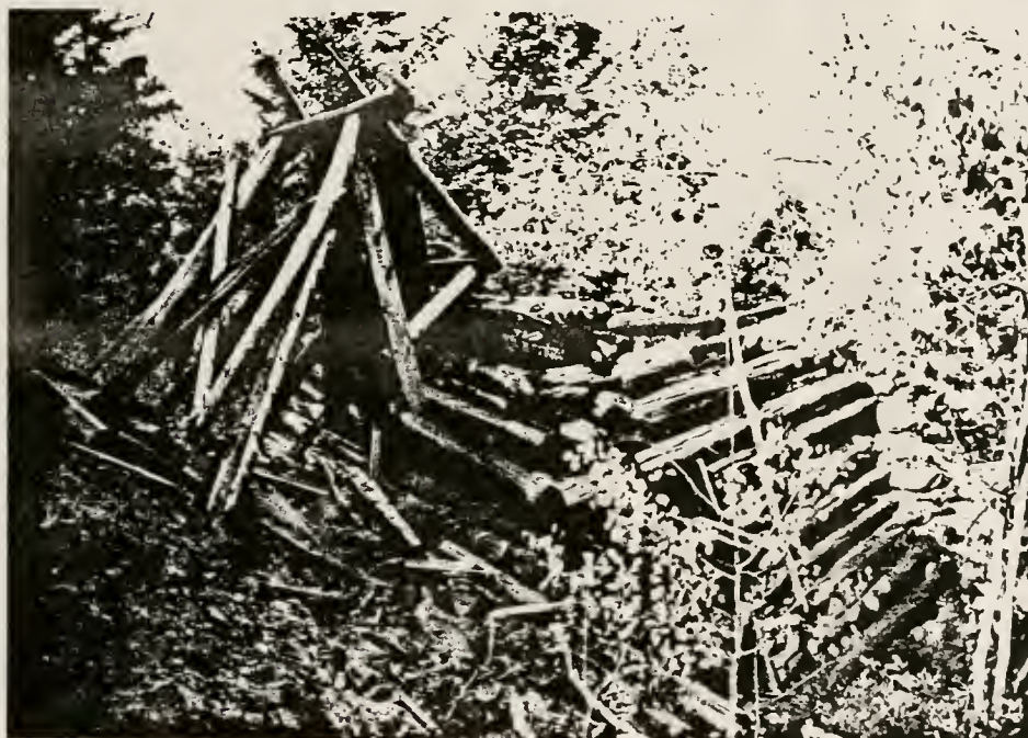
Figure 246. Feature #139, log ore bin, southwest view.
